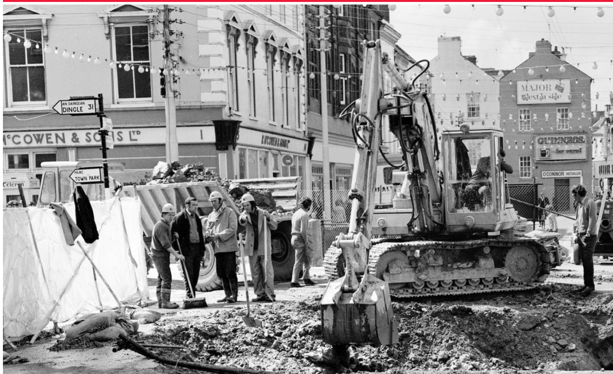
Castle Street, Tralee, during the construction of the culvert in May 1974
